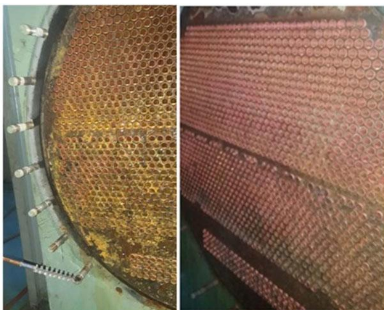
Condenser Tube Cleaning
