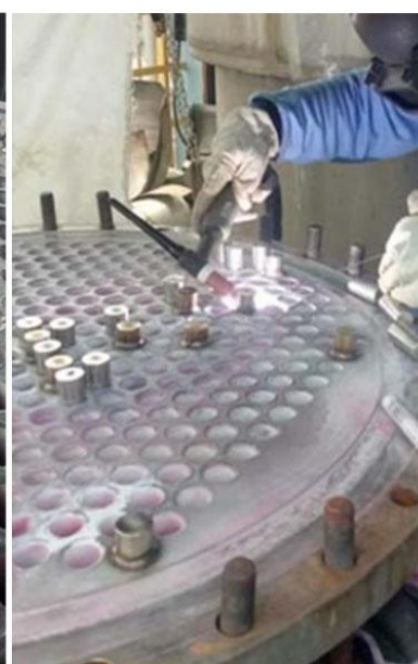
Repair Heat Exchanger & Plug Tube
