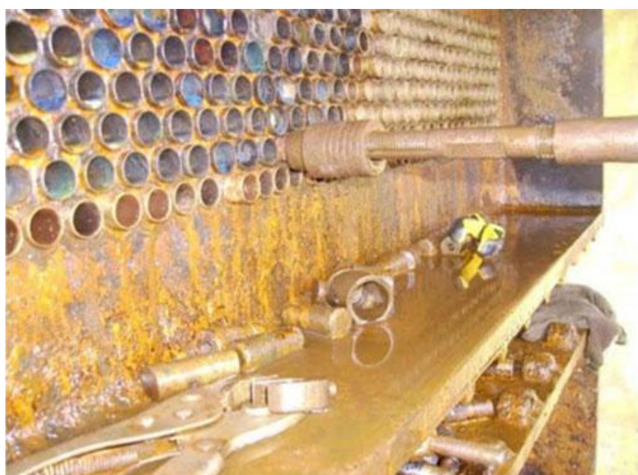
Re-tubing Heat Exchanger
