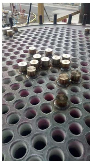
Repair Heat Exchanger & Plug Tube
